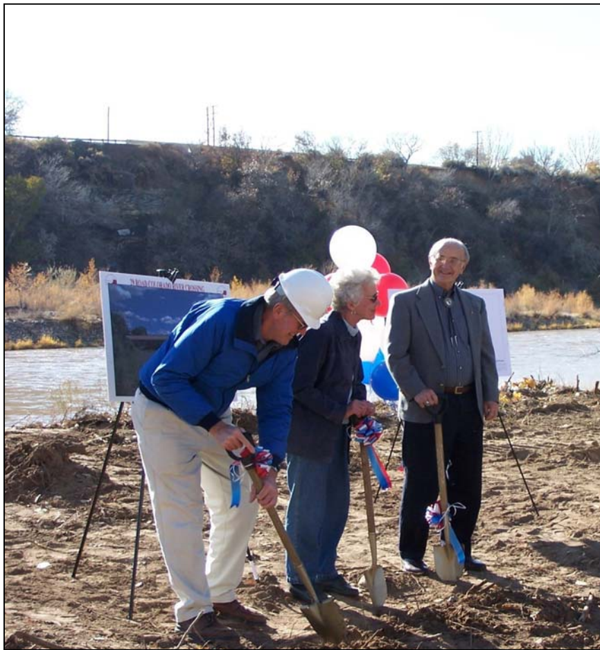
The Board of County Commissioners (From left to right: James R. Baughman, Tilman M. Bishop and Doralyn B. Genova) at the ground breaking ceremony on November 10, 2004 for the 29 Road Bridge over the Colorado River. The Bridge is anticipated to be completed by October 2006.
