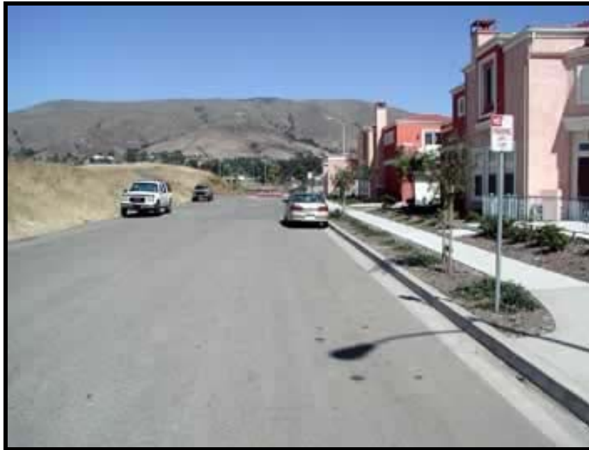
Source: www.pedbikeimages.org/Dan Burden
