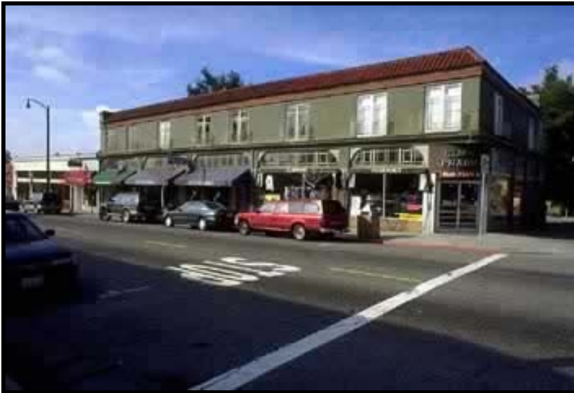
Source: www.pedbikeimages.org /Dan Burden
