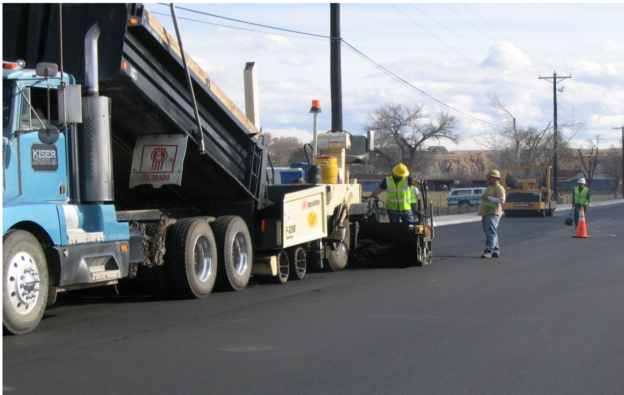
Construction of 33 Road
