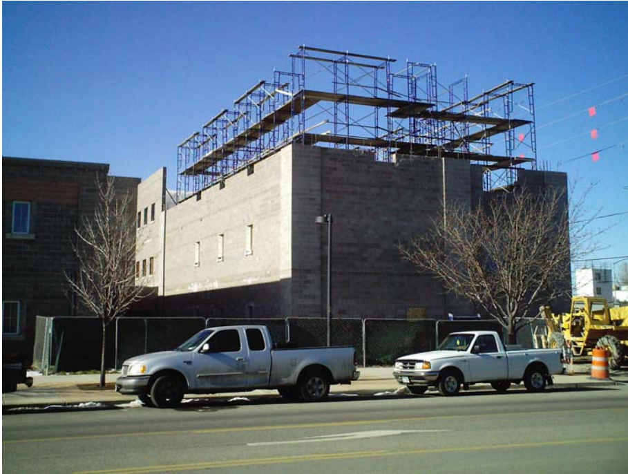
Construction of the Community Corrections & Methamphetamine Treatment Center
