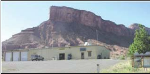
Figure 1: Gateway Community Center
