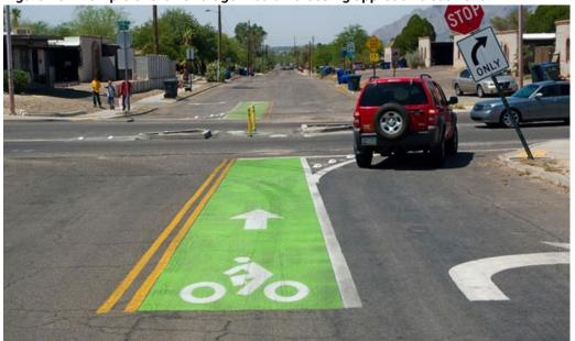
Figure 16. Example of a bike refuge median crossing approach treatment.
