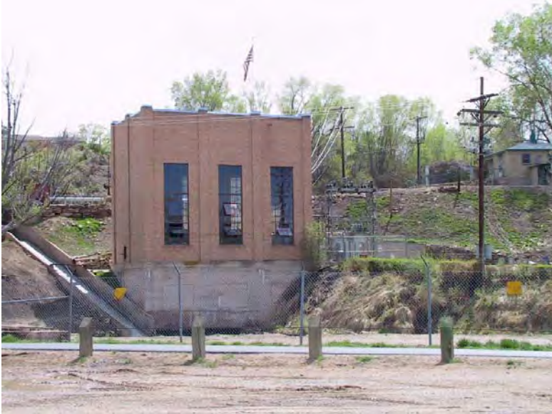
Redlands Power Canal and Power Station
